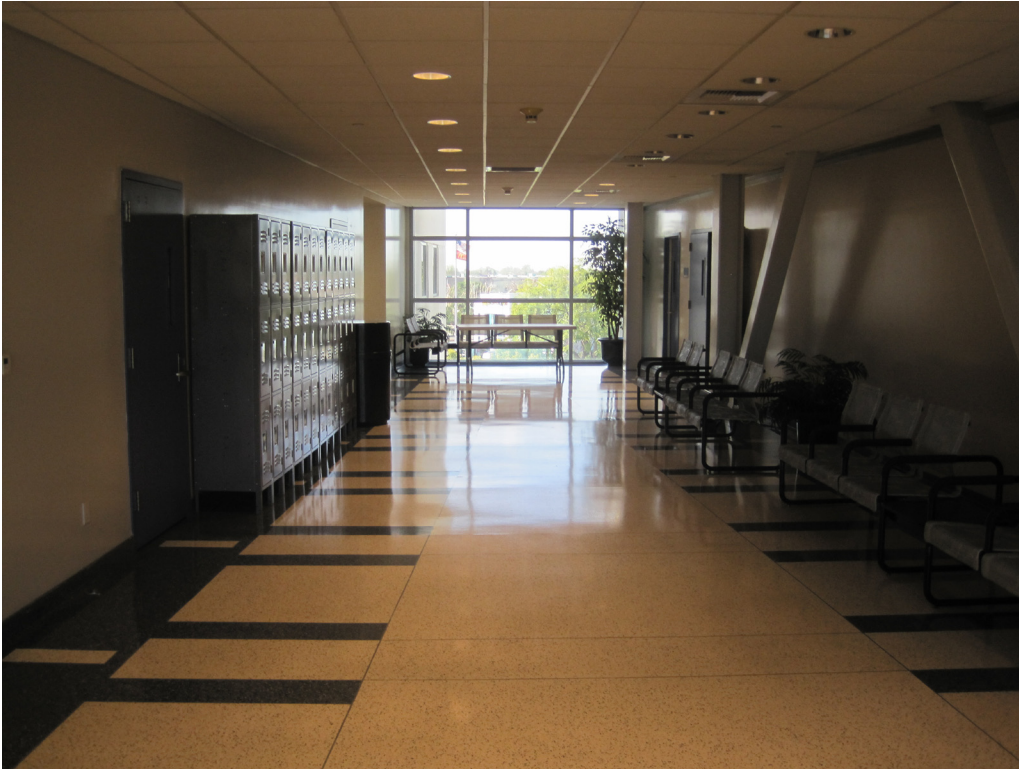
Existing Corridor Conditions
